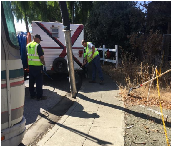
Staff using a vacuum truck to clean an illicit RV discharge. Image courtesy of City of Mountain View.
